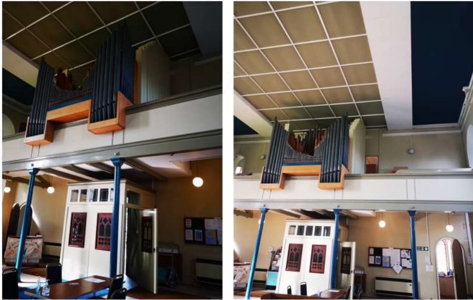
Photo No A5 - North/ south bays and mezzanine level in the West end of church
