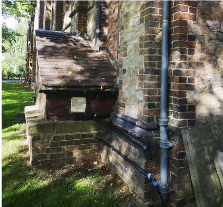
Image 3 – Diagonal cracks in basement staircore
