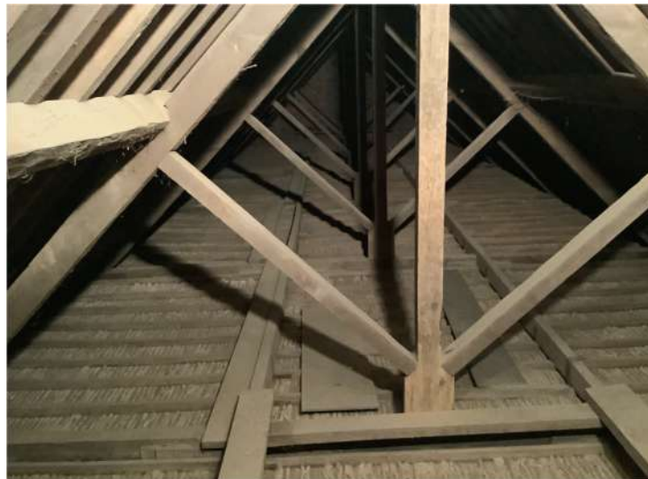
Photo A4- Historic photo of Roof Truss
