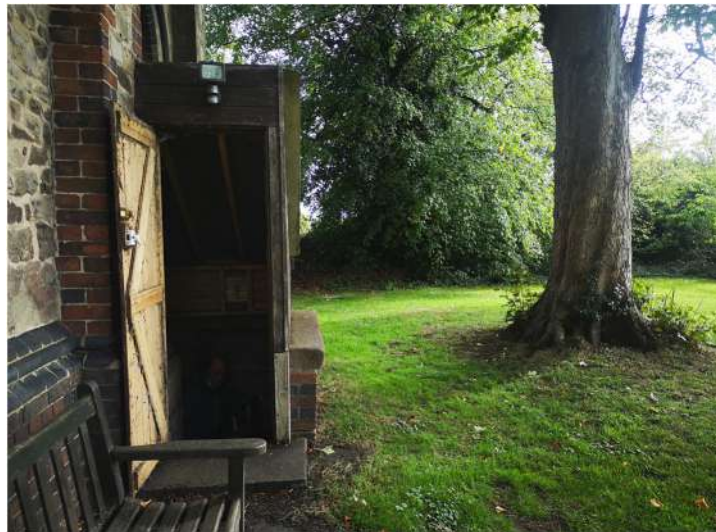
Photo A6 Basement doorway at the South East side of Church
