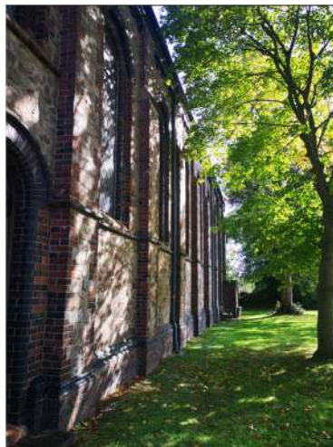
Photo A2- South Elevation wall showing nearby trees
