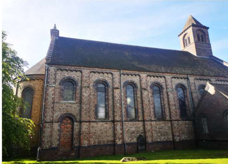
Photo A3- North Elevation view
